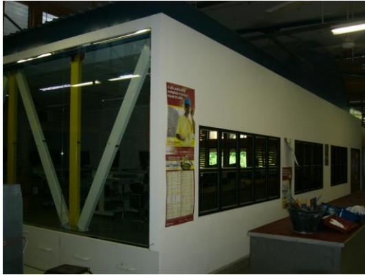
Figure 1 External appearance of the “Structural Learning Space”
